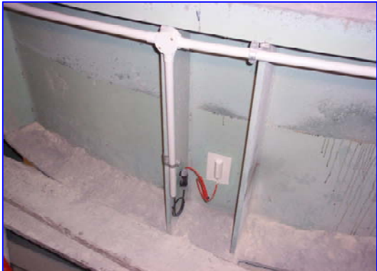
Silo-weigh is successfully monitoring contents of huge 500 tonne silos at Pilkington Glass in St Helens, Lancs
