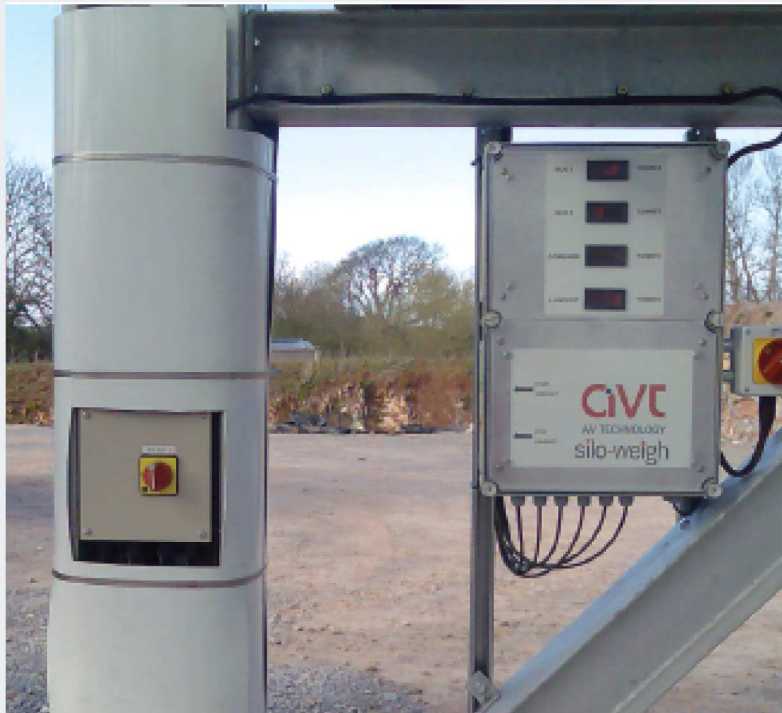
The AVT central control and readout unit
